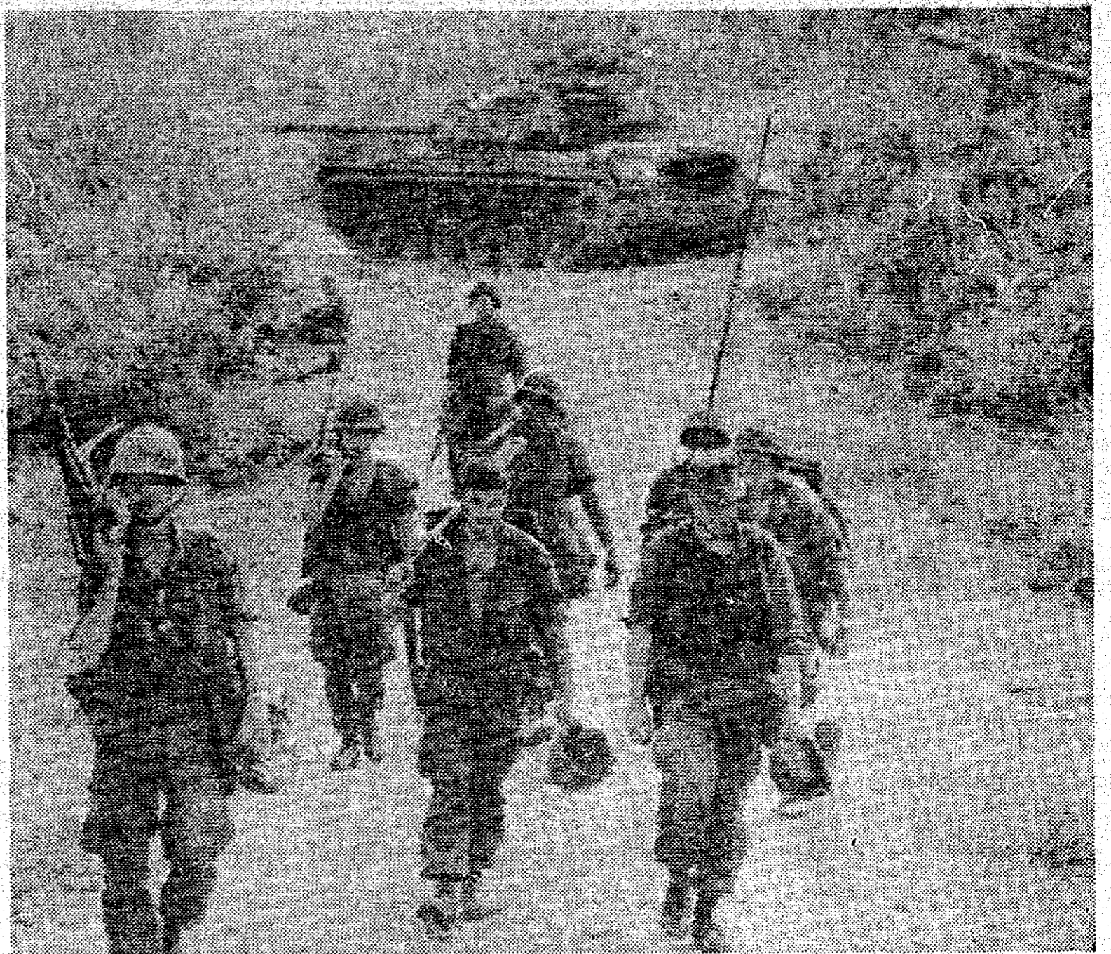
A squad of U.S. Marine engineers moves up Route 9 toward Khe Sanh during the lifting of the siege at the Marine combat base. The long-closed road was being repaired. (AP Radiophoto)
