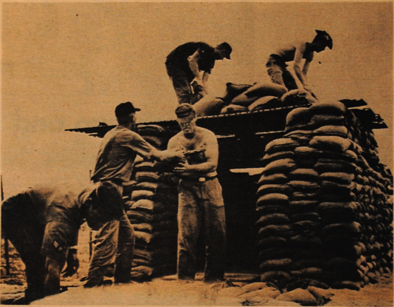
Men of the 1st MOB team in Vietnam pile sandbags on a bunker to house some of their communications equipment. MOB has special
