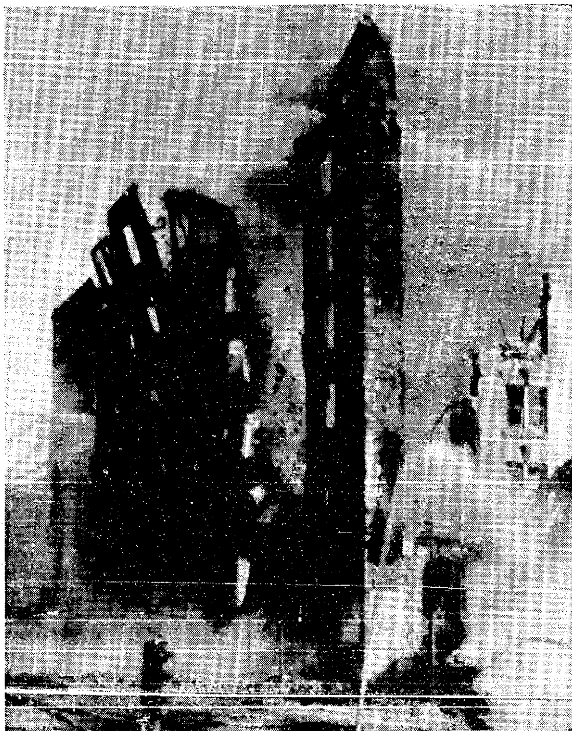
WALLS OF THE FIRE-SWEPT NORMANDIE HOTEL IN PHILADELPHIA CRUMBLE
